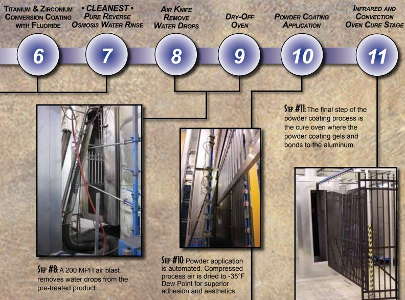
STEP **#9**: A convection oven completes the dry-off process.
